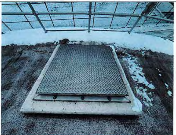
Exterior roof hatch #2
