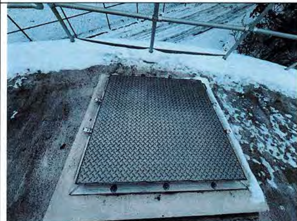
Exterior roof hatch #1
