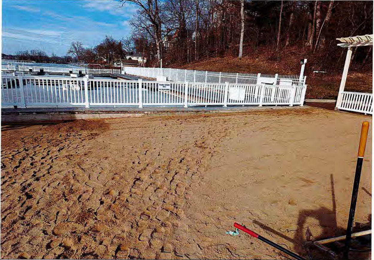
Initial Beach and Dock Restoration
