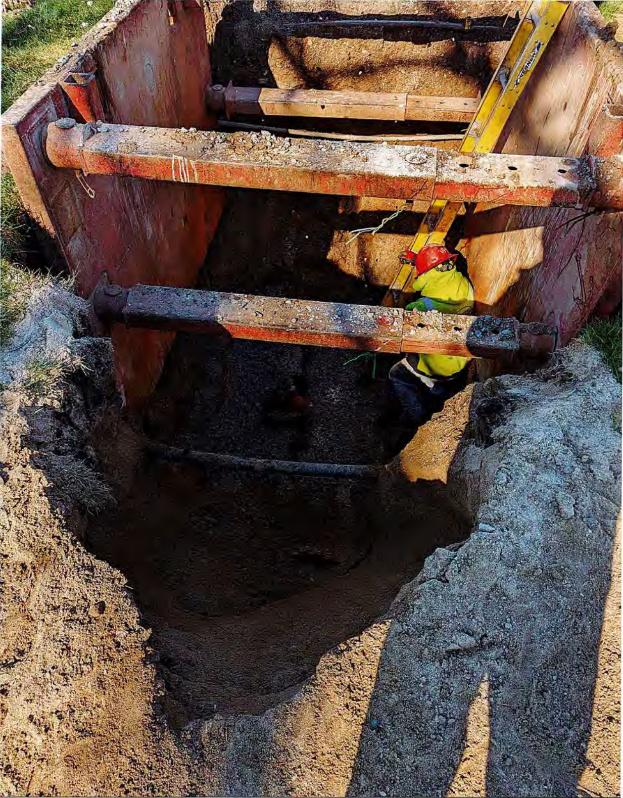
New 8-Inch Valve Installed on Watermain Leading to Clubhouse
