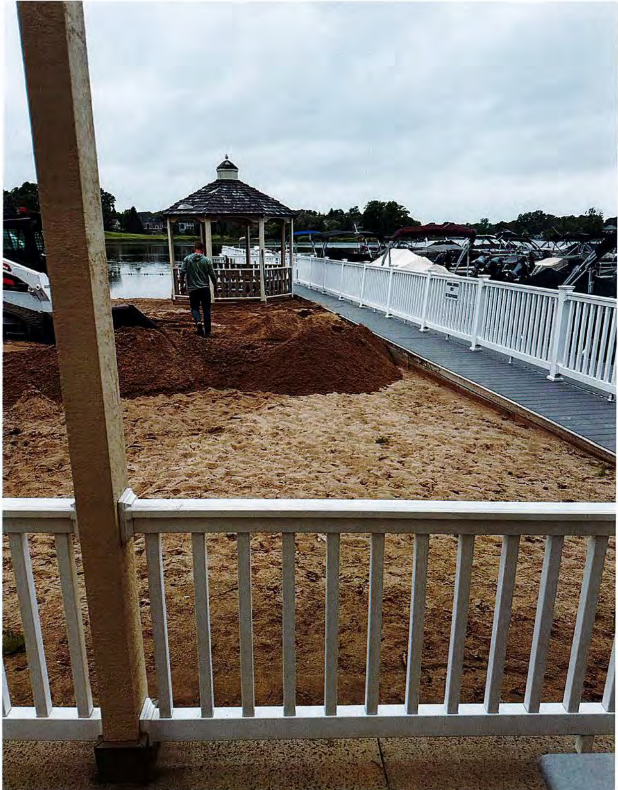
Additional Beach and Dock Restoration
