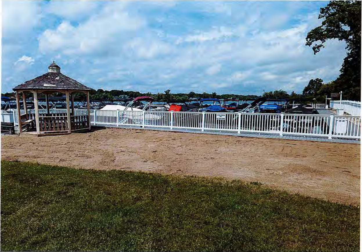
Final Beach and Dock Restoration
