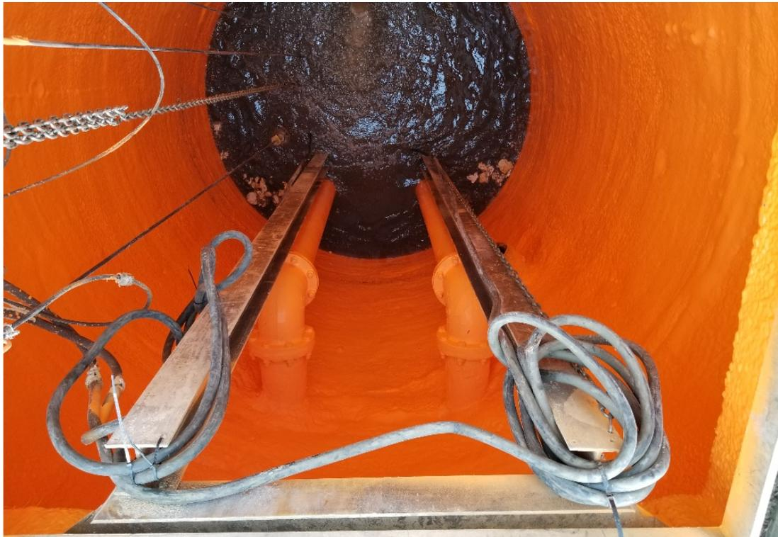
Picture 7: OBIC Lining of Pump Station 11, Coating of Concrete and Piping
