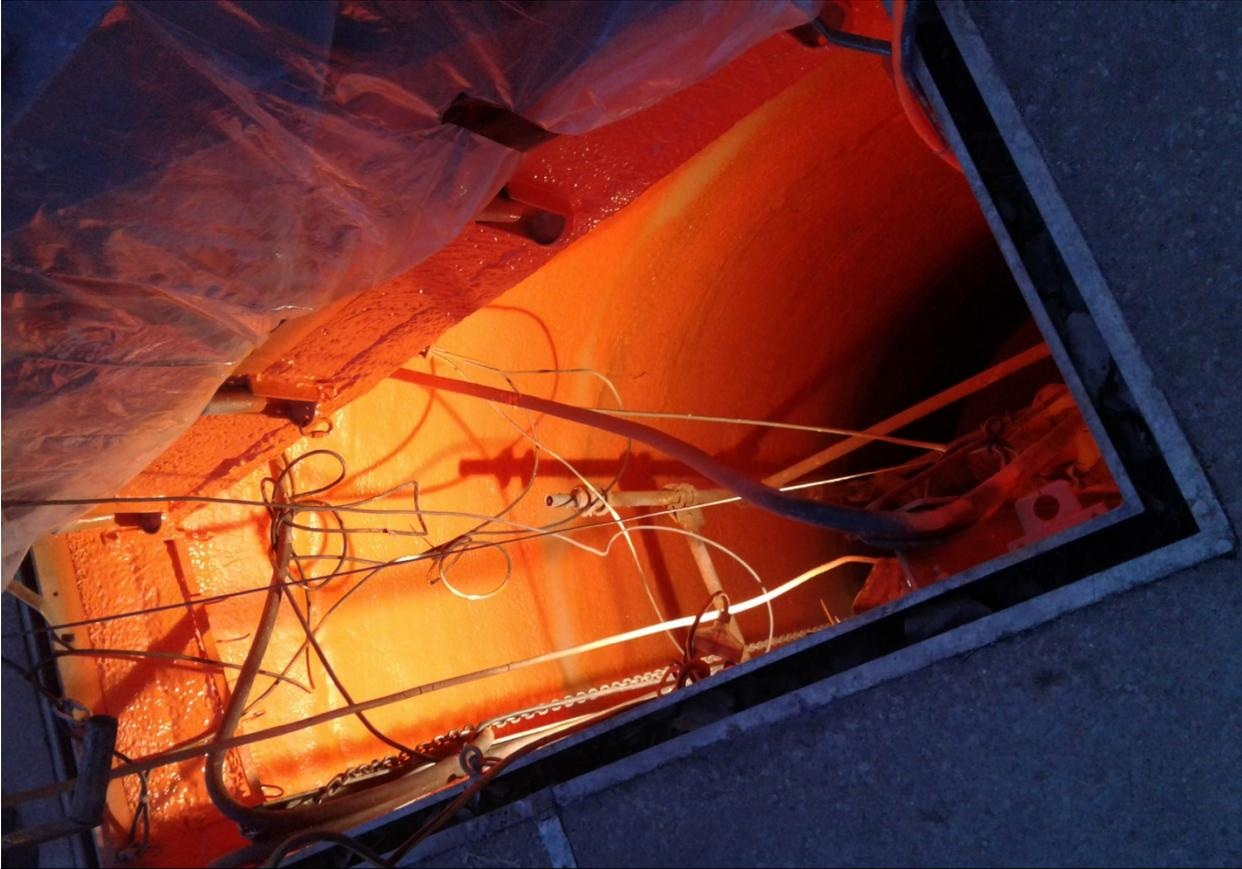
Picture 8: OBIC Lining of Pump Station 06, Coating of Concrete and Piping
