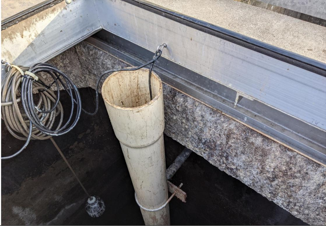
Picture 4: Concrete Corrosion Near Level Transducer on EQ Tank 3
