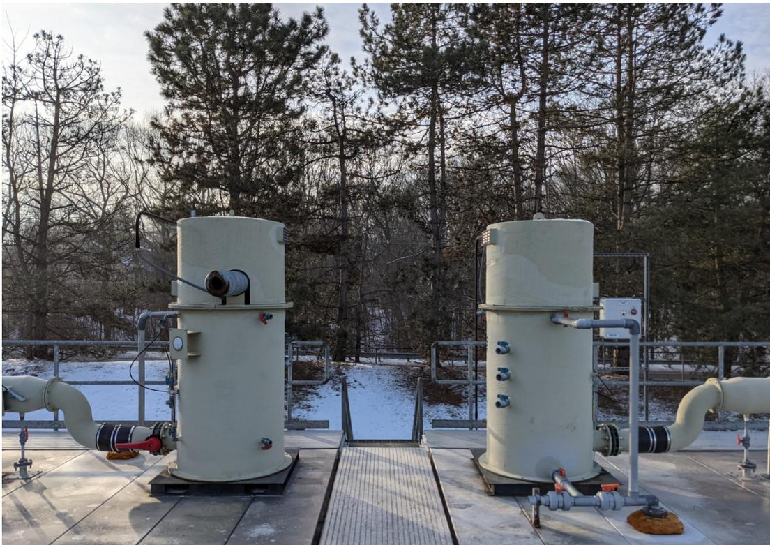
Picture 2: Aluminum Covers Over Primary EQ Tanks 2 and 3, Carbon Odor Control System
