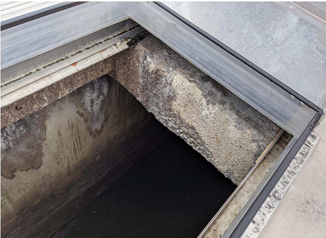
Picture 5: Concrete Corrosion on Cross Beam and Walls on EQ Tank 2
