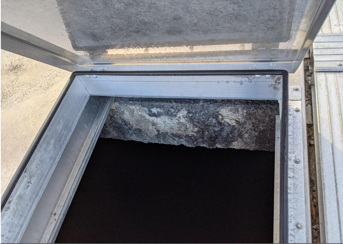
Picture 6: Concrete Corrosion on Cross Beam in EQ Tank 3
