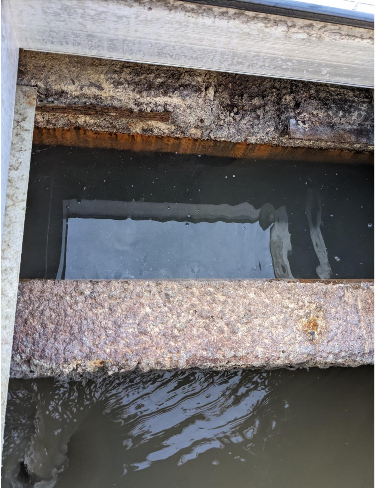
Picture 3: Concrete Corrosion in Influent Channel, Note Reinforcing Steel Protruding on South Wall
