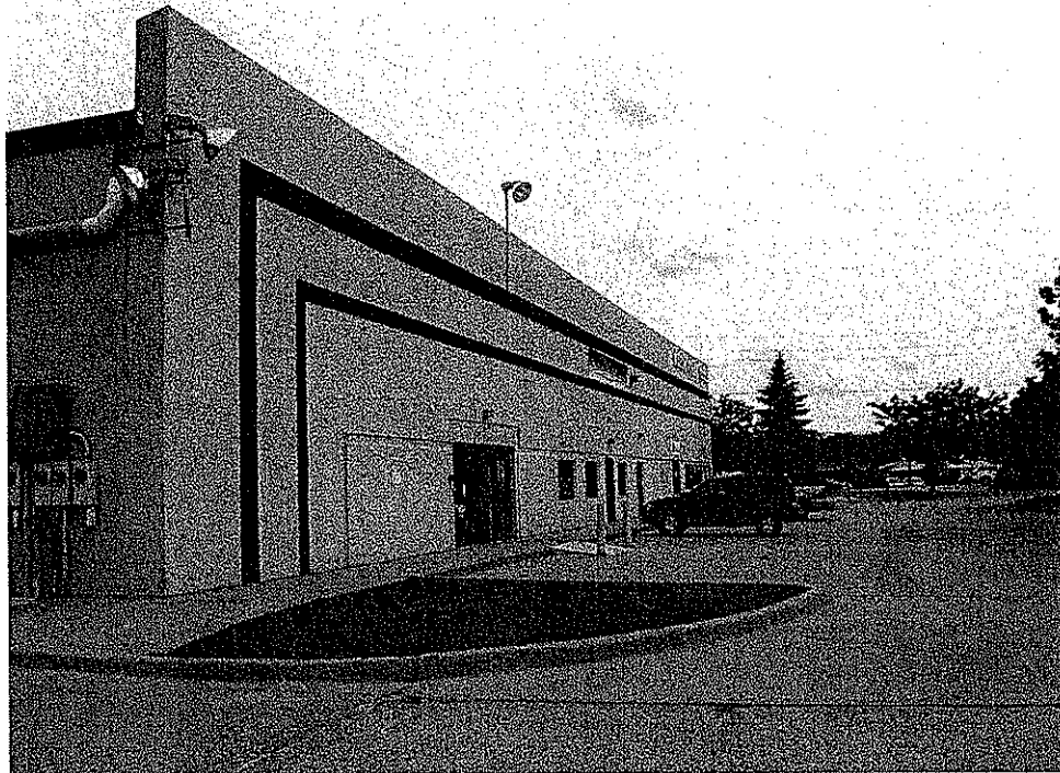
NORTHWEST CORNER OF BLDG.- SIDE ELEVATION OF THE WELL † INSIGHTS (WALL SIGN FOR THE WELL TO REPLACE JOHN DEERE) NO OTHER FACADE CHANGES PROPOSED
