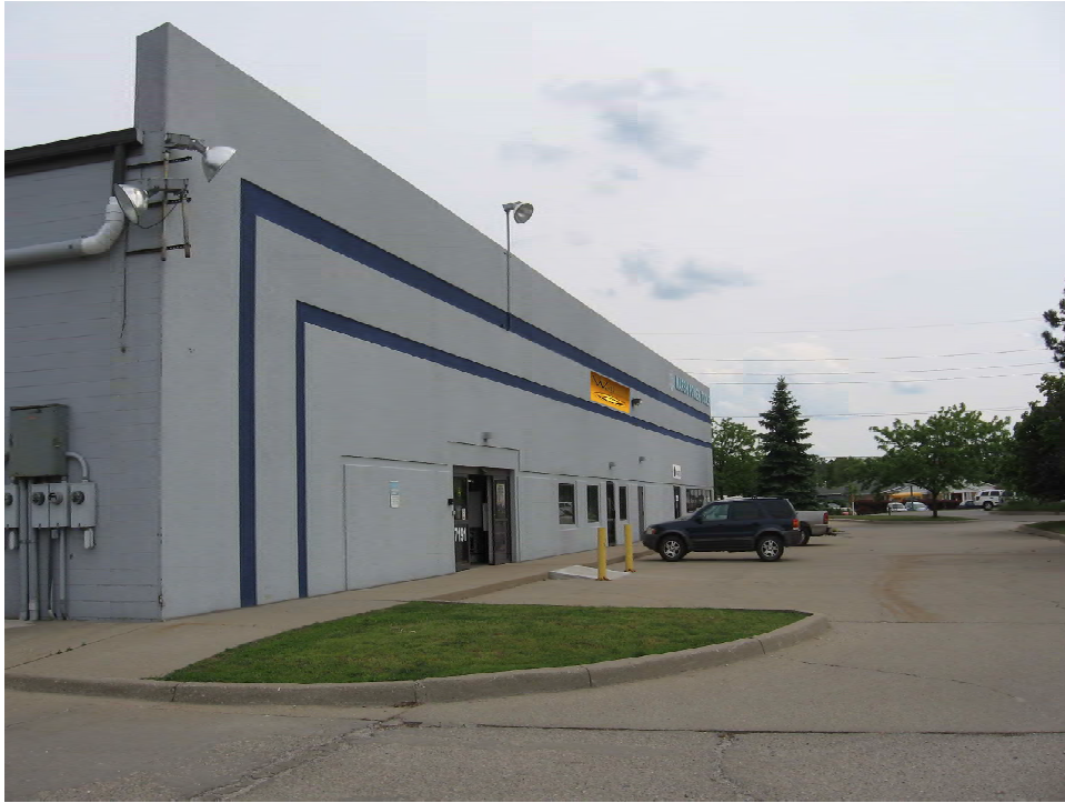
NORTHWEST CORNER OF BLDG.- SIDE ELEVATION OF THE WELL & INSIGHTS (WALL SIGN FOR THE WELL TO REPLACE JOHN DEERE) NO OTHER FACADE CHANGES PROPOSED
